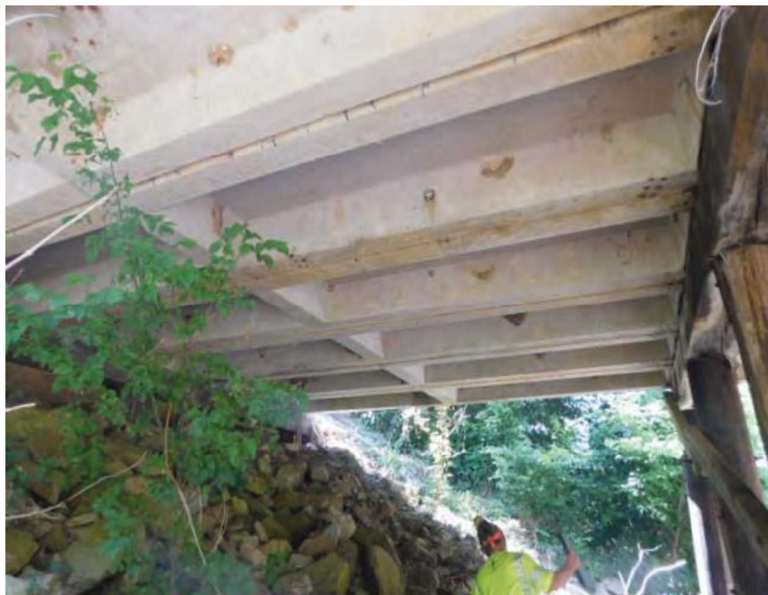
BOTTOM DECK SPAN 3
