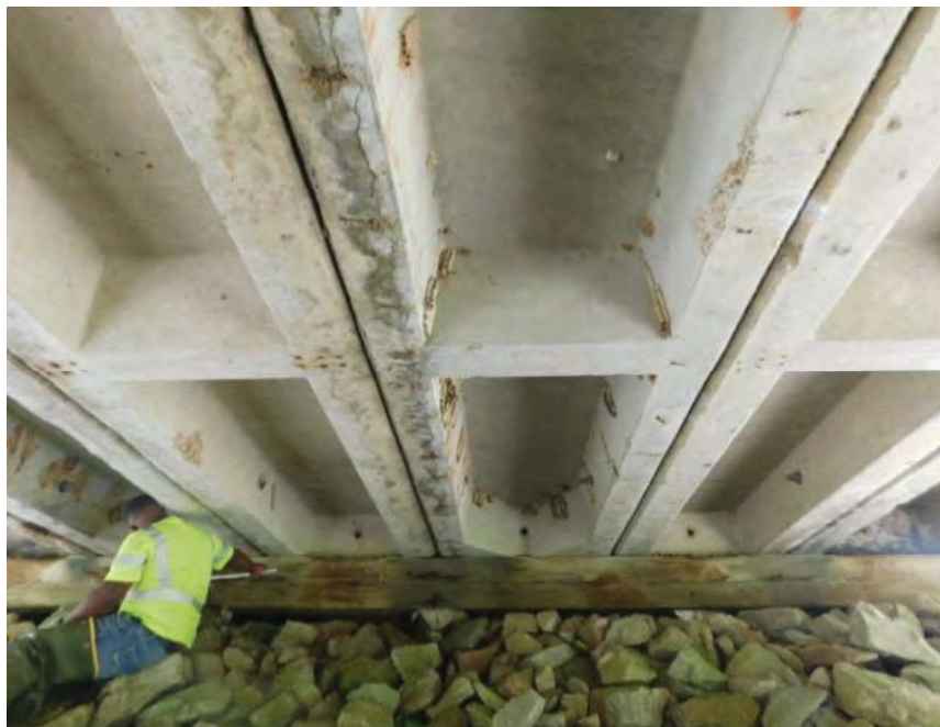
BOTTOM DECK SPAN 1
