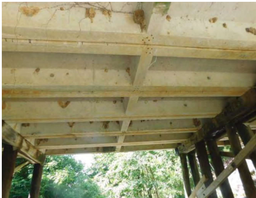
BOTTOM DECK SPAN 2
